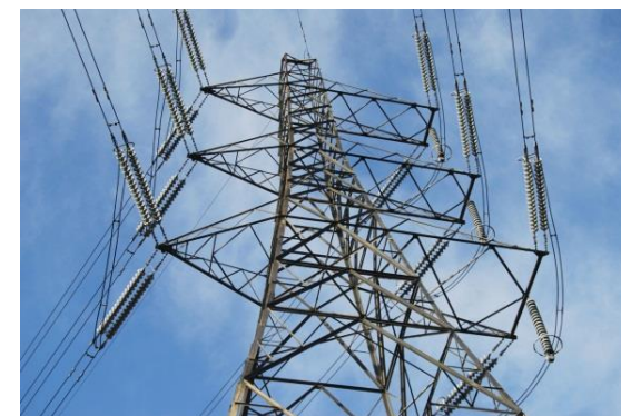
Overhead power lines
